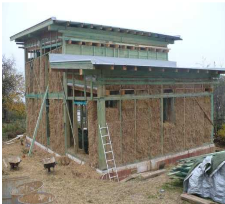
Fig. 2: Example of a straw house in a structural system with a non-load-bearing straw "two by four". By author.
