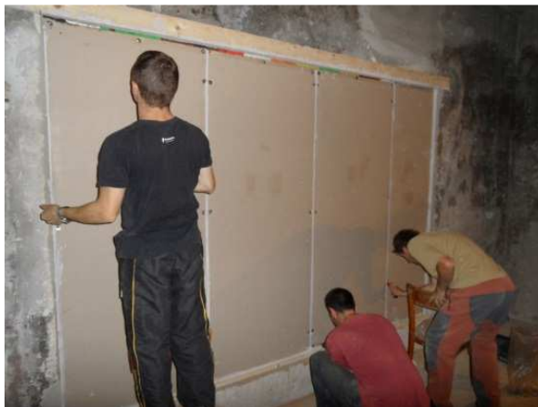
Fig. 10: Assembly and sealing of the gaps of additional Ecopanel s wall. By author.
