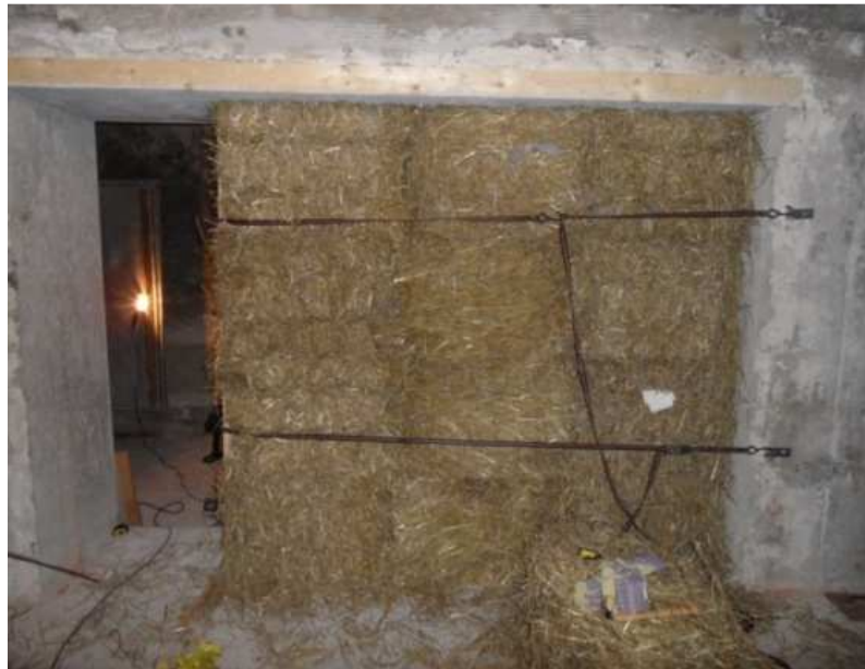
Fig. 3: Gradual assembly of the straw wall into the test hole in the acoustic laboratory chamber of Brno University of Technology. By author.
