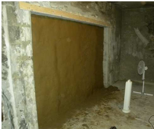
Fig. 5: Drying-out of external clay plaster before measurement. By author.
