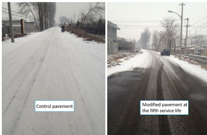
Figure 10. A section of the road in Beijing of China.
