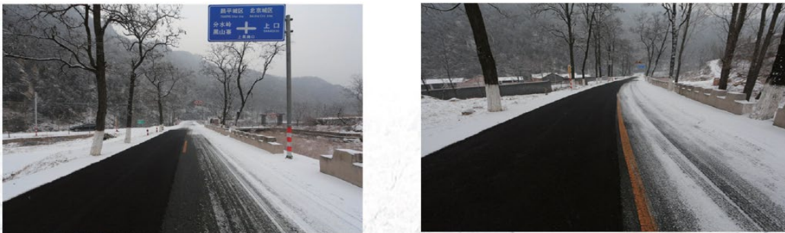
Figure 9. A section of the road in Beijing of China.
