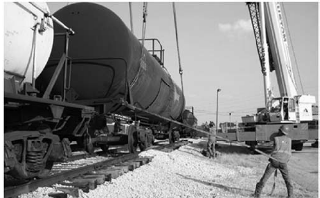
Decatur Memorial Hospital donated a railcar for use in HazMat training.
