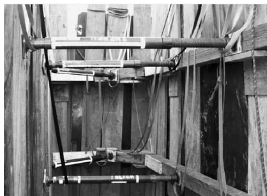
Down in the trench prop.
