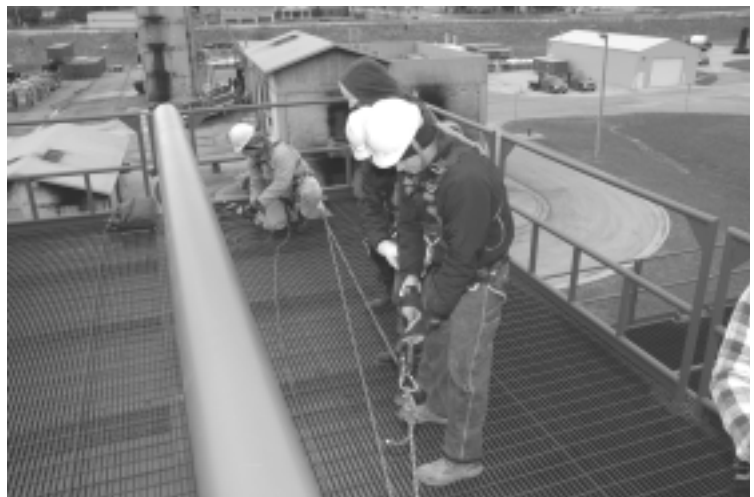
Confined Space Technicians checking a haul system prior to using it to remove a victim.
