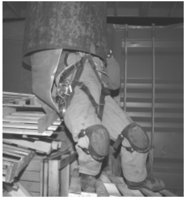
Vertical entry into a confined space with collapse and entrapment of a victim using a supplied air respirator.
