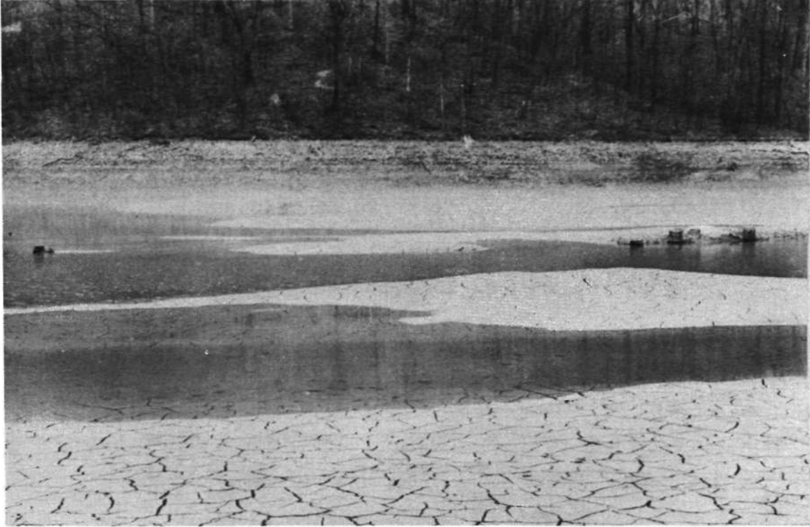
Figure 6. Sediment Deposit on Reservoir Bottom.
