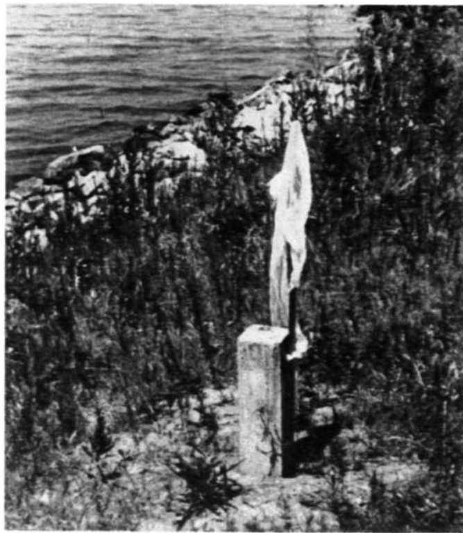
Figure 4. Concrete Post Used to Mark Survey Stations.
