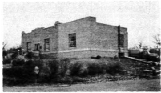
FIG. 9. WEST FRANKFORT WATER TREATMENT PLANT.
