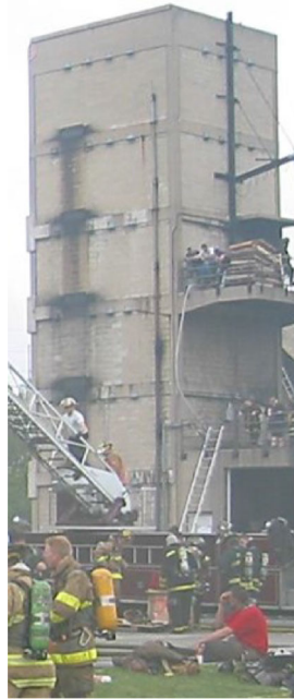
(a) Northeast corner of Structure B
