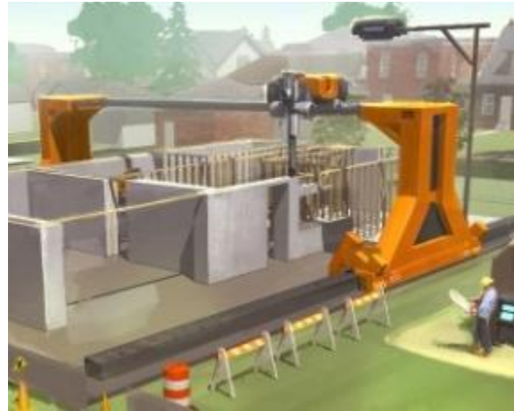
Figure 2.10.1: Use of CC to Build House dailytrojan.com
