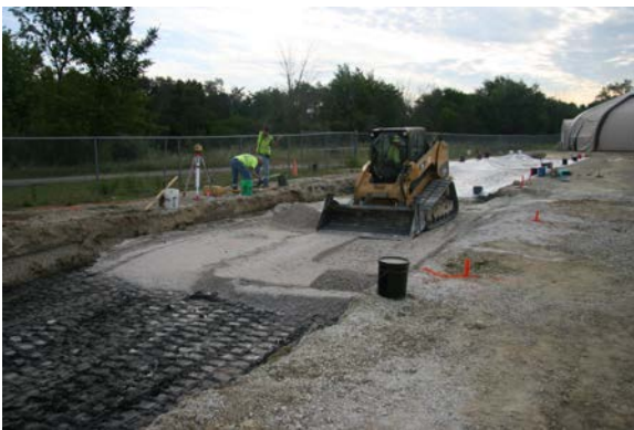
Construction of C1S4 unbound layers
