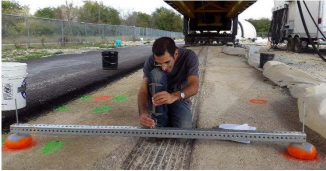
(a) Customized Rut Depth Measuring Device
