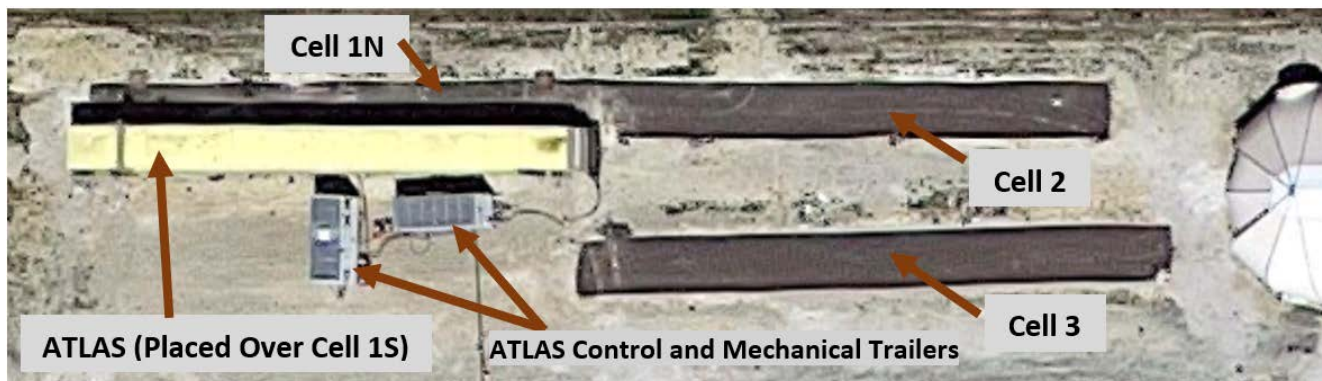
Figure 4.1. Google satellite view of the construction site showing overall the constructed test cells.
