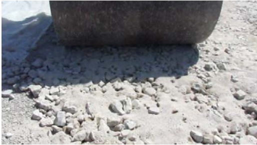
QB1 placed on top of PCR (before compaction)
