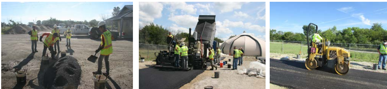
Figure 4.15. Hot mix asphalt sampling and paving.
