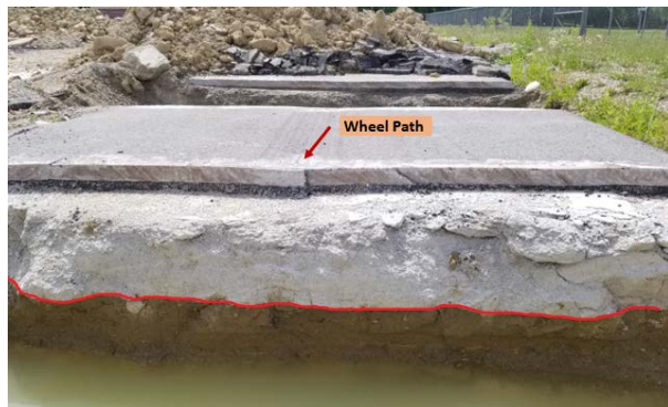
C2S4W – QB2 + Cement
