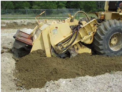
Subgrade Soil Tilling and Mixing
