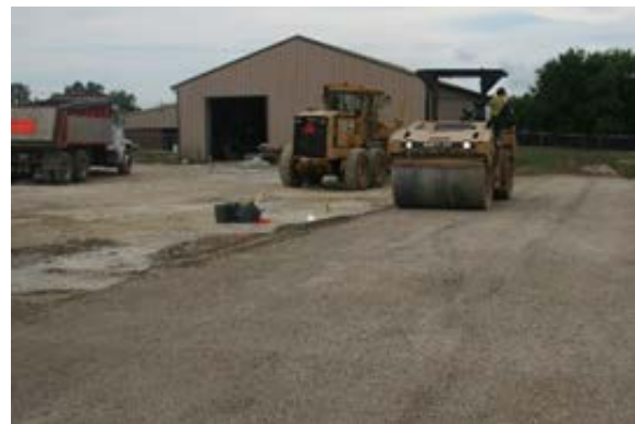
Placement of CA06_R Capping layer for Cell 1
