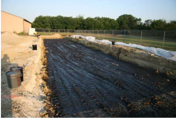
Subgrade Surface after Application of Tack Coat
