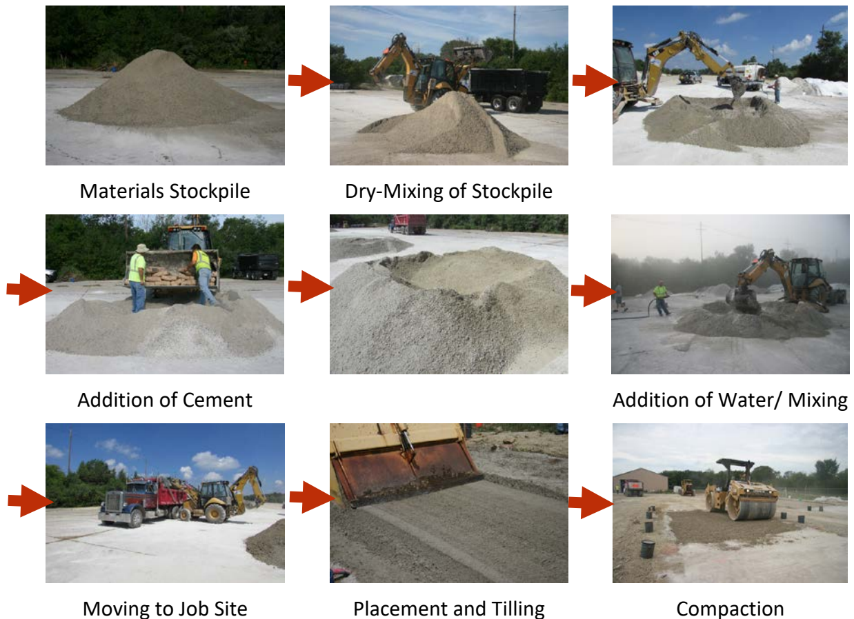
Figure 4.13. Construction of chemically stabilized test sections in Cells 2 and 3.
