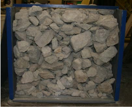
Aggregate subgrade compacted in two lifts
