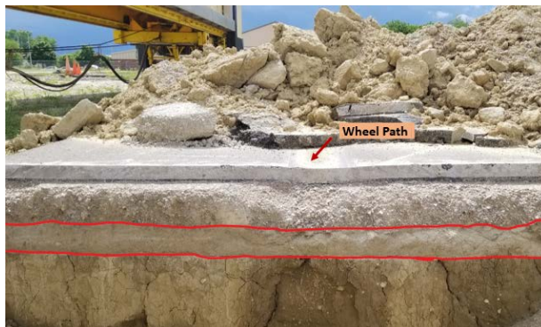
C3S3W – QB2 + Fly Ash Subbase & CA06_R Base
