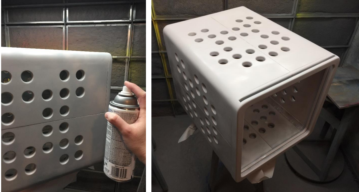
Figure 4.14: Applied primer, sanded and spray paint
