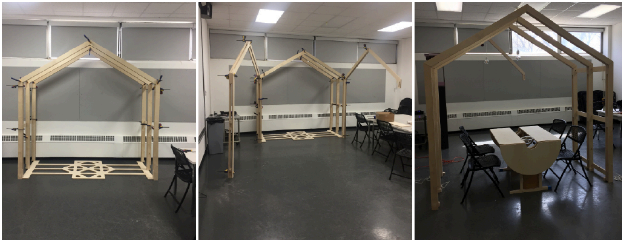
Figure 4.1: After designing the pieces in CAD, all structural elements were cut on the CNC out of \frac{3}{4} " Baltic Birch Plywood. These images show the dry-fit assembly of the final prototype in various stages.
