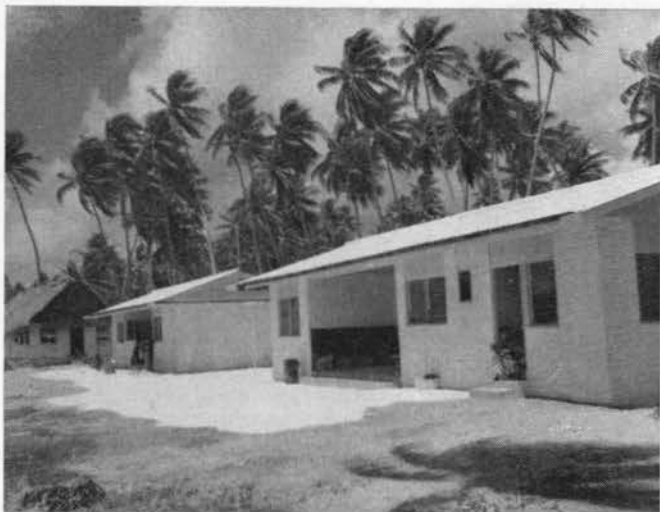
The Assistant Medical Officer on Penrhyn Island lives next door to his work. The farther of the two concrete buildings is the A.M.O.'s house, and the nearer is the island dispensary.
