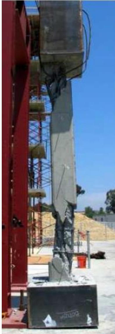
Figure 5.72. Test 8- post-test, removed from fixture [17]
