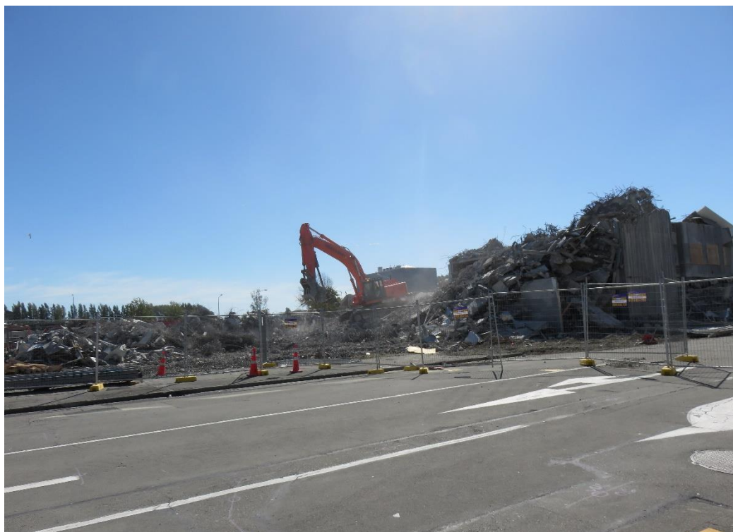
Figure 10: Demolition work in the city centre
