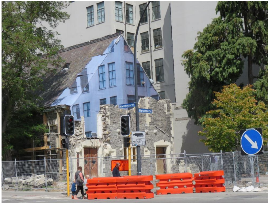
Figure 2: Building works in Christchurch's city centre
