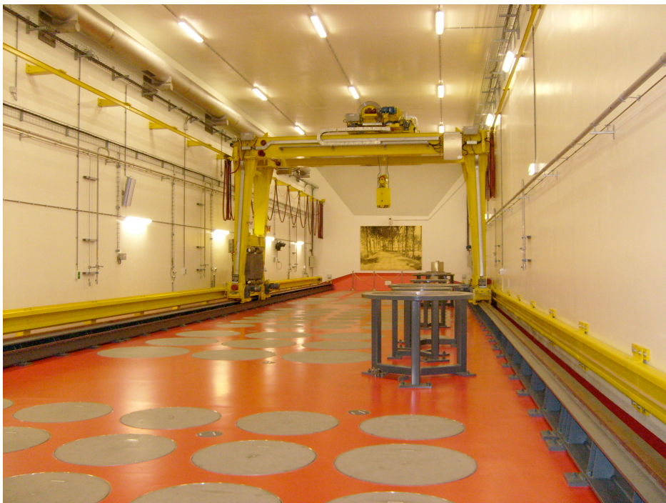
Figure 3. Nuclear waste storage in the Netherlands. Circles on the floor marking the presence of nuclear waste. Creative Commons.
