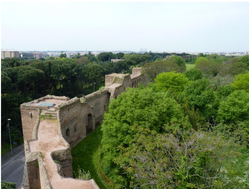
Fig. 2.8 A stretch of the Aurelian Wall at the Porta Appia .
