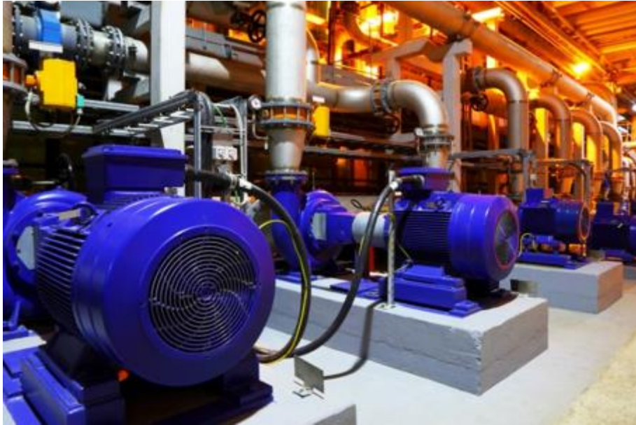
Figure 2-7 Centrifugal pump in water pumping station [62].
