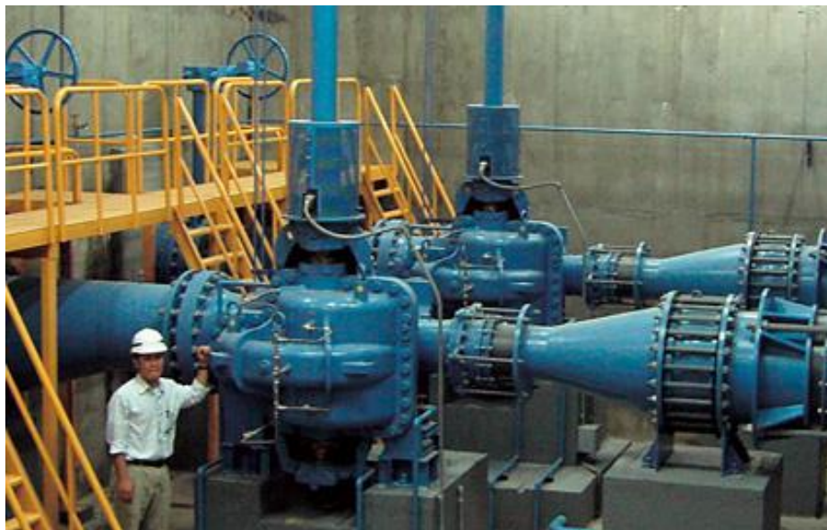
Figure 2-6 Centrifugal pump in a water treatment plants [61].
