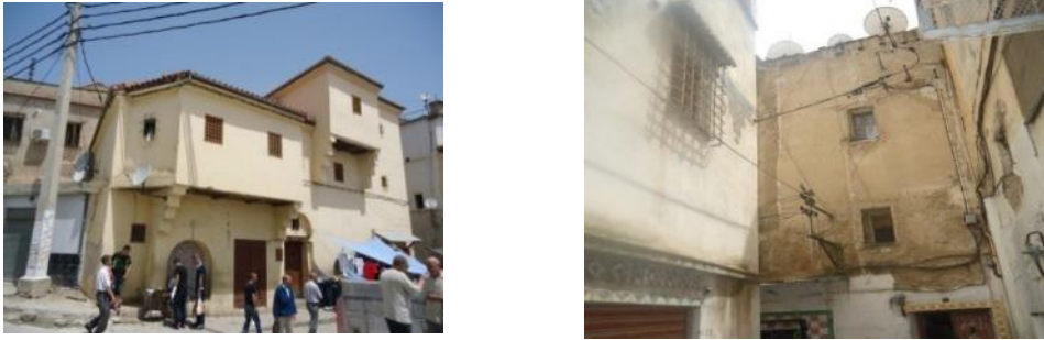
Figure 6.31: Security Measures - Iron grids: A) Interior facades and B) Exterior facades.
