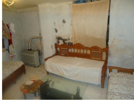
Figure 8.1: The use of heaters.
