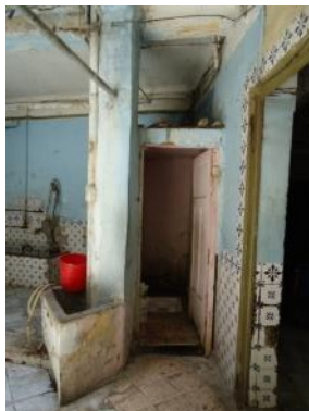
Figure 7.3: A case study house with a shared toilet.
