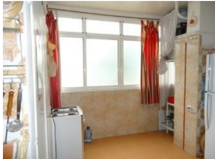
Figure 7.33: Closed loggia in 400 houses estate.
