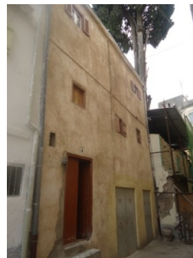
Figure 8.7: Small exterior windows
