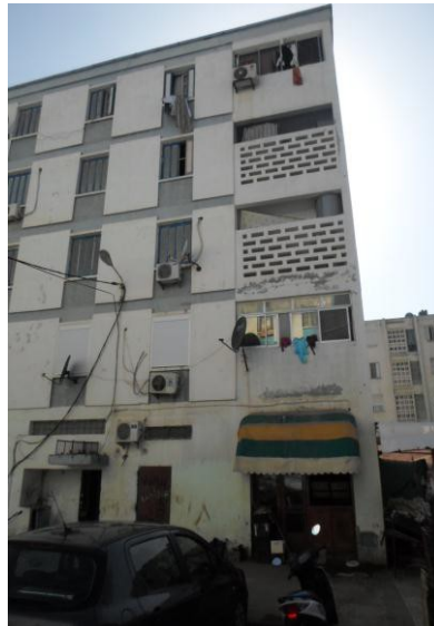
Figure 3: Example of ‘closed’ balconies
