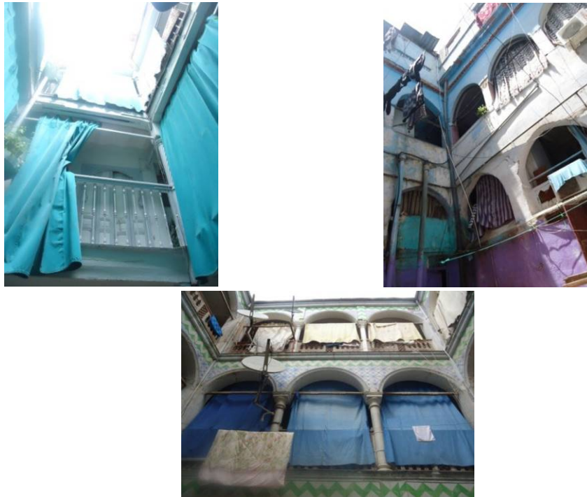
Figure 8.8: The use of curtains as a protection from sunshine.
