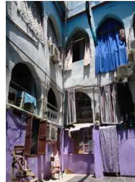
Figure 8.2: The use of air conditioners.
