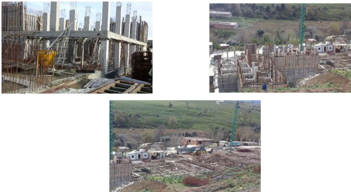
Figure 3.5: The project of 280 LPP houses in Jijel (January 2016).
