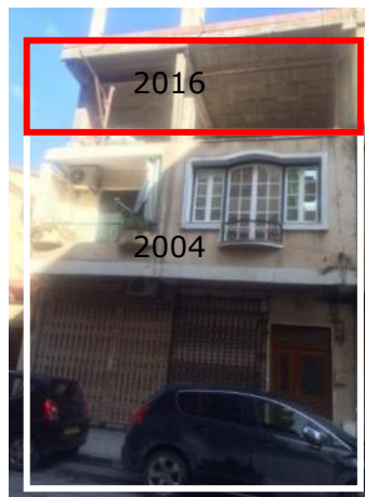
Figure 6.8: Continuing work in an individual house.
