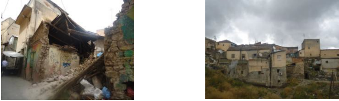
Figure 6.10: Demolished houses in Souika.
