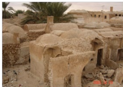
Figure 4.8: Ruined traditional house in Oued Souf (Belhadj, 2007).
