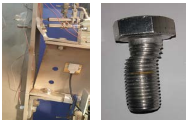
(b) TSAC-O-10 connection failure mode and deformed top bolt with crack initiation
