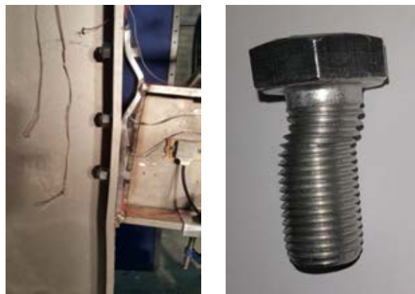
(b) Extended End Plate (EEP-O) connection failure mode and deformed top bolt
