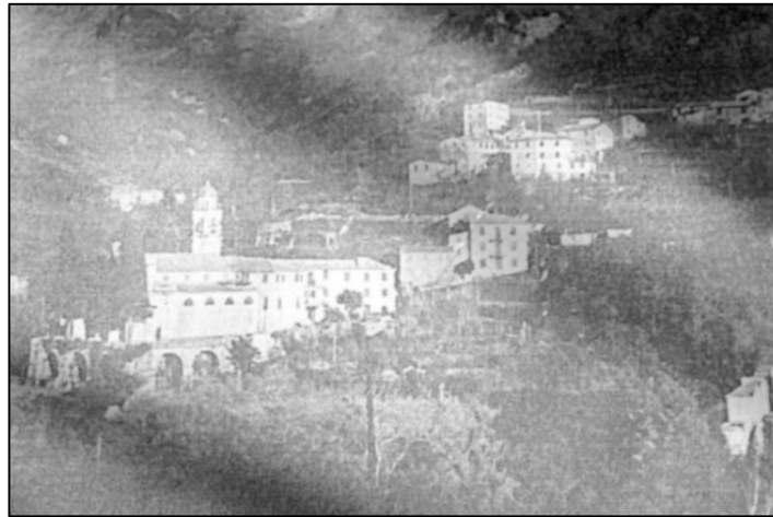
4.21. View of Monteghirfo, 1990s
