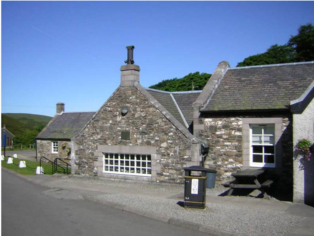
Museum of Lead Mining, side elevation from car park
