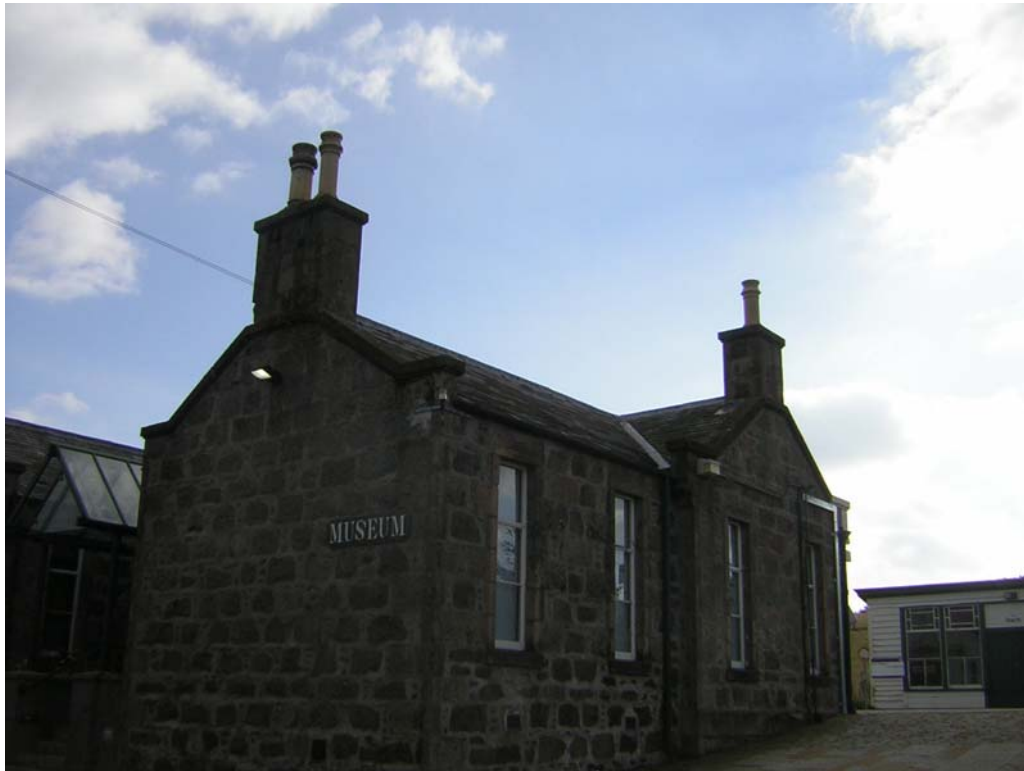
Insch Connection, viewed from railway station car park
