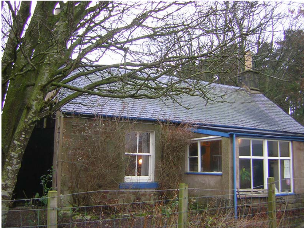
Brownsbank Cottage, view of front elevation
