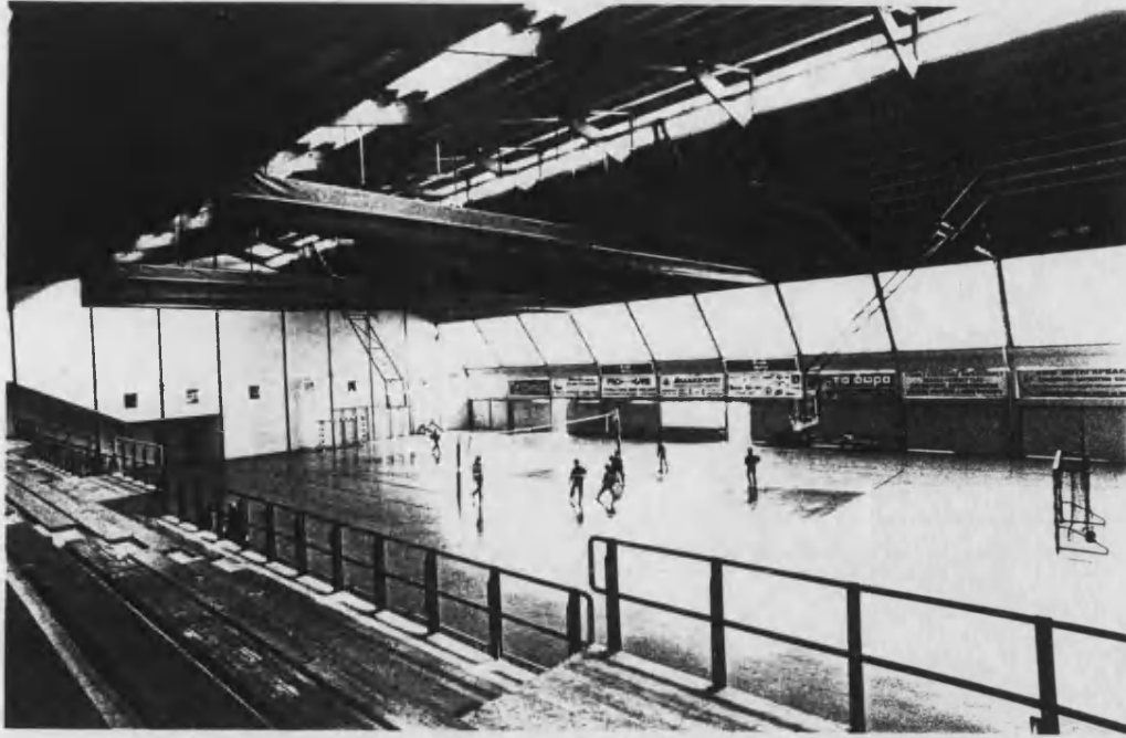
Figure E.13 Interior View of Loutraki Sportshall from the Seating Area (note two sources of natural lighting, north windows and north rooflight)
