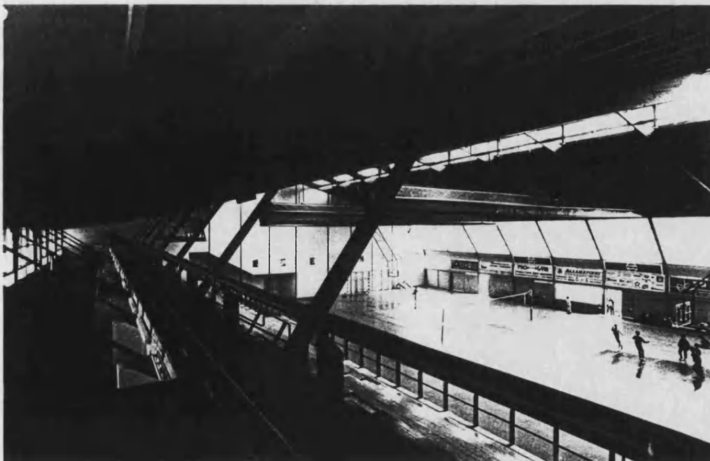
Figure E.12 Interior View of Loutraki Sportshall from the Seating Area (high contrast between natural lighting in seating versus playing area)
