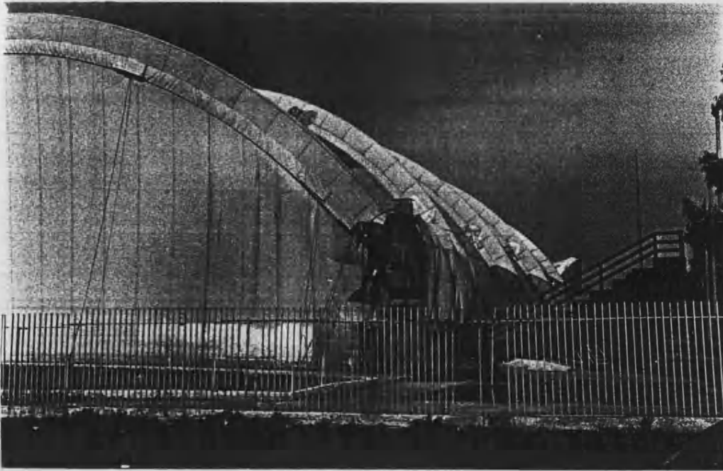
Figure E.8 South East View of Patra Swimming Pool
