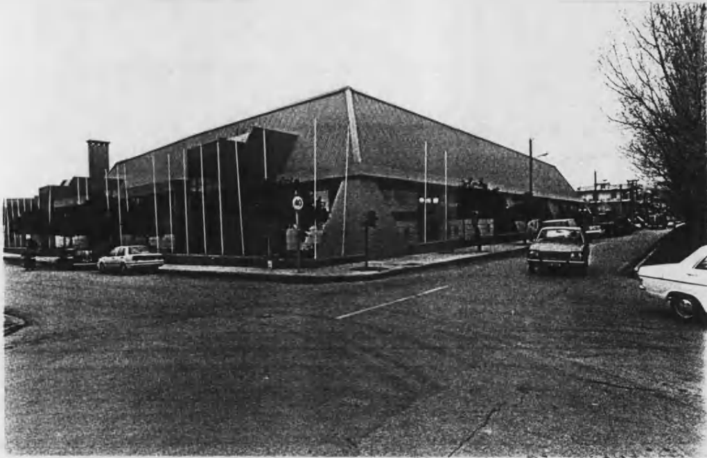
SOUTH WEST VIEW
