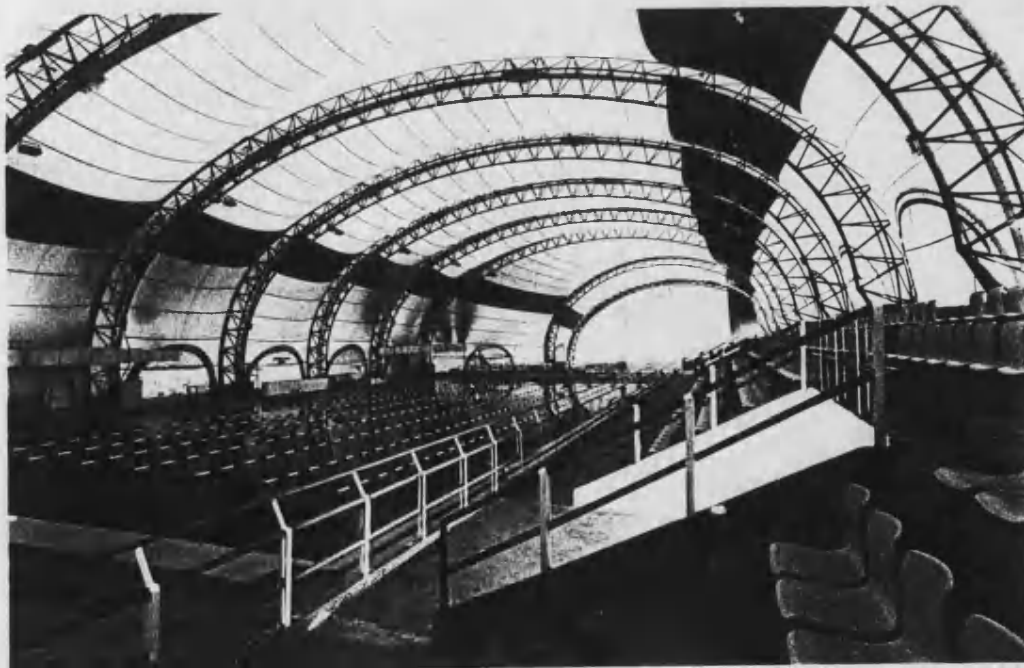
Figure E.14 Daytime Interior View of Posidonio Swimming Pool
