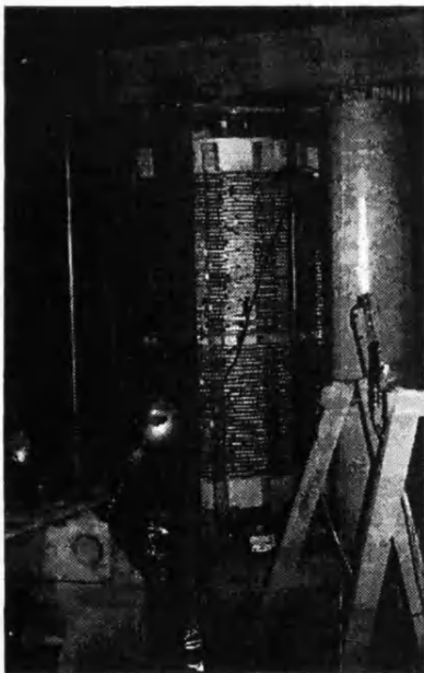
Fig. 3. Transformer winding used for generating discharge sources
