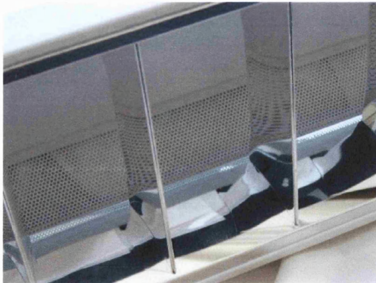
Figure 5.13: The luminaires used in the test room. They included mirrored reflectors to limit glare and a perforated casing to allow a proportion of light to be directed upwards.
