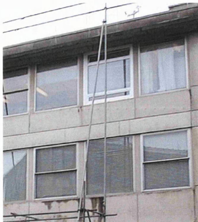
Figure 5.7: A photograph showing the new window in place.
