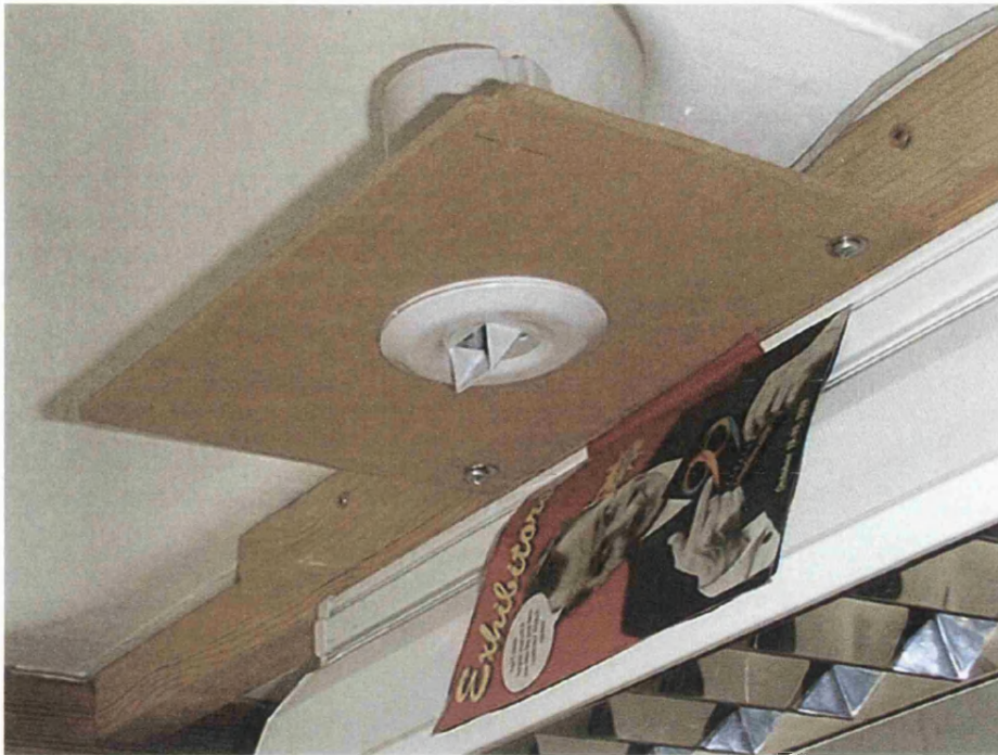
Figure 5.15: The shield window sensor, or angle sensor. Unfortunately the shielding was not totally successful as the hole in the casing for the service LED let light through to the sensing element. This affected the control of the lights so as a result a piece of paper was fitted to shield the sensor from the direct light from the lamp.
