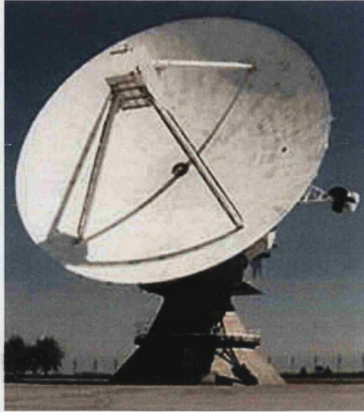
Figure 3.8: The Chilbolton Advanced Meteorological Radar (CAMRA) with its 25 m antenna.
