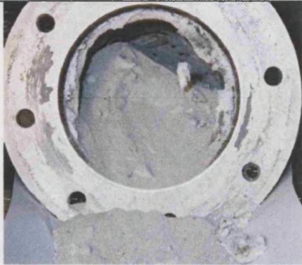
Figure 4.56 Run 4: Combustion Tube at ignitor.
