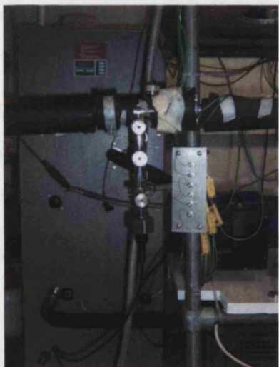
Figure 3.2.3: Closer look at T-piece including thermocouples.
