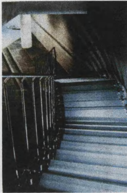
Figure 1.6 A cantilevered glass staircase at the Pilkington research and development headquarters in Lathom, John Colvin, Pilkington Architectural, 1996.
