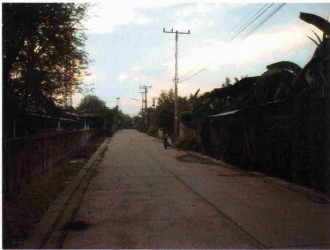
Figure 5.5: Concrete road in Ban Lao Source: Own Photograph (2005)
