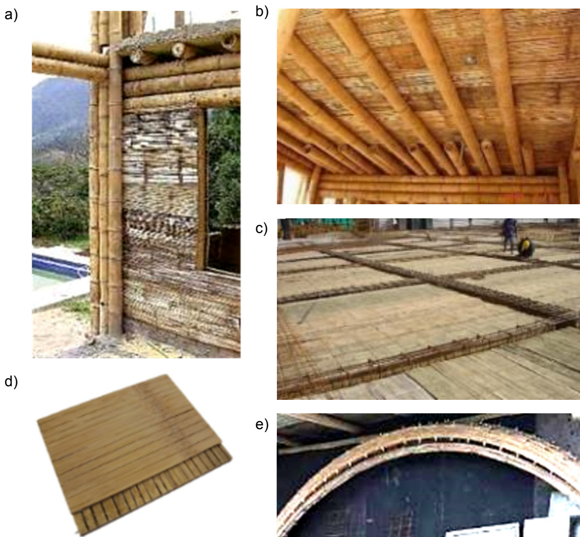
Figure 3-3. Riven Guadua uses in construction. a) Wall sheathing, b) Roof & Ceilings, c) Floors, d) Slab formwork and (e) Arc configuration.
