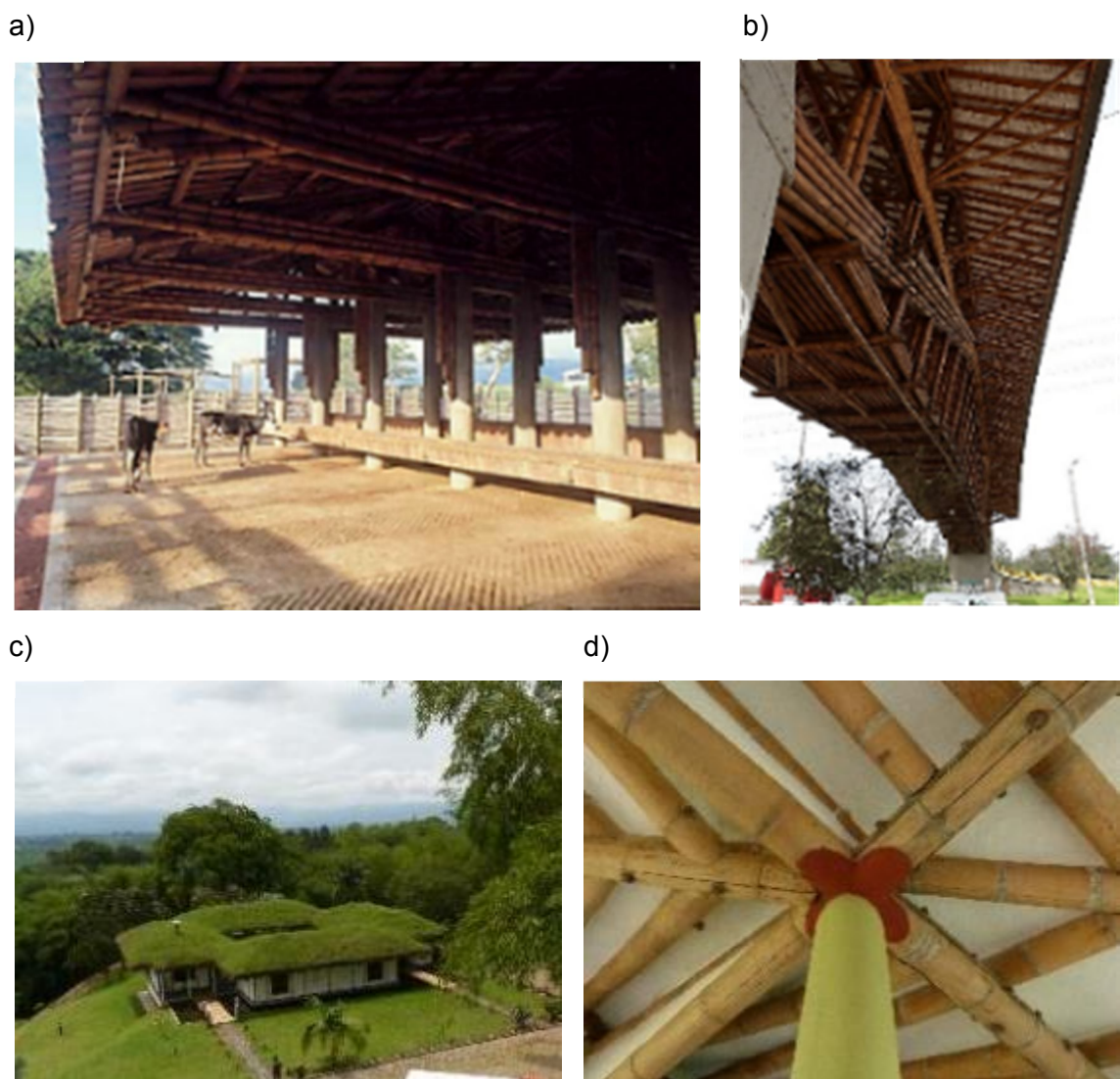
Figure 3-7. Bamboo buildings using Guadua by Simón Vélez in Colombia. a) Cantilevered roof of a stable by Simón Vélez (Villegas, 1989). b) Forty-meter span pedestrian bridge in Bogotá. c) Holiday house in the coffee growing region and d) Roof structure detail.
