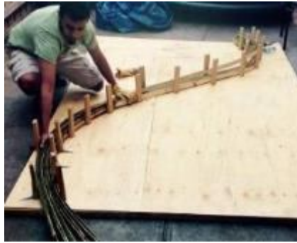
Figure 11-13. Bamboo bent for the roof structure of a tent ( http://www.giantgrassdesign.com )
