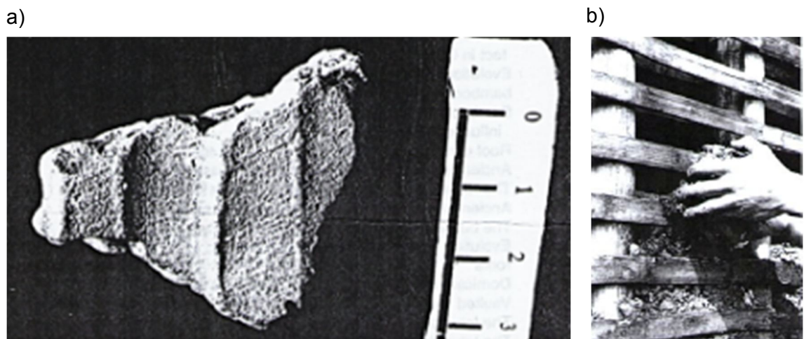
Figure 3-4. a) 3,500 years old Fossilized clay with bamboo slats impressions. b) Wattle and daub technique - bahareque (Hidalgo-López, 2003)
