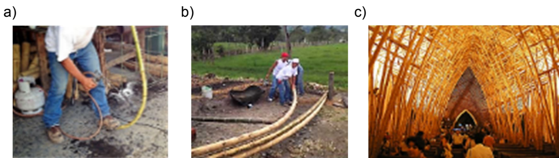
Figure 4-3. a) Bending round bamboo with a gas flame burner. b) Bending green Guadua by manual force ( www.guaduaibamboo.com ). c) Bent Guadua construction temporary built in Pereira after the 1999 earthquake in Colombia.
