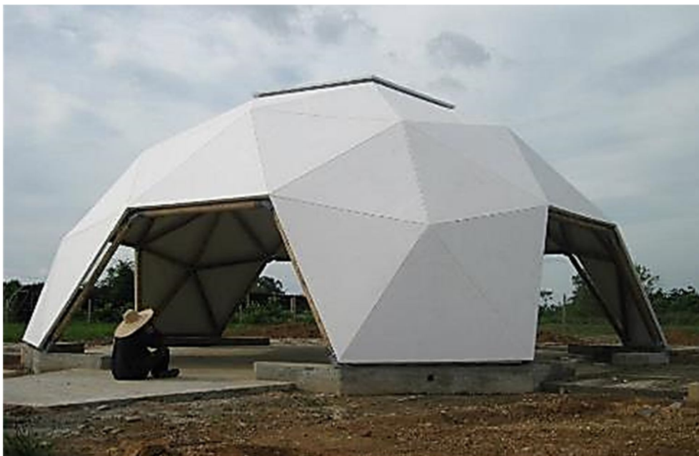
Figure 3-17. Stainless steel connections. a) German-Chinese House at Expo-Shanghai 2010 ( www.in-habitat.com ). b) Connections and domes by Guaduatech (Guaduatech Inc.)
