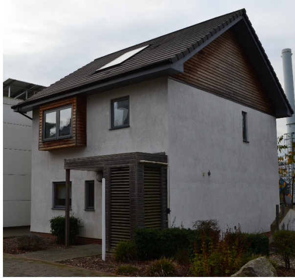
Figure 1.3: The renewable house, showcase hemp-lime walled three bedroom house, Building Research Establishment, Watford.
