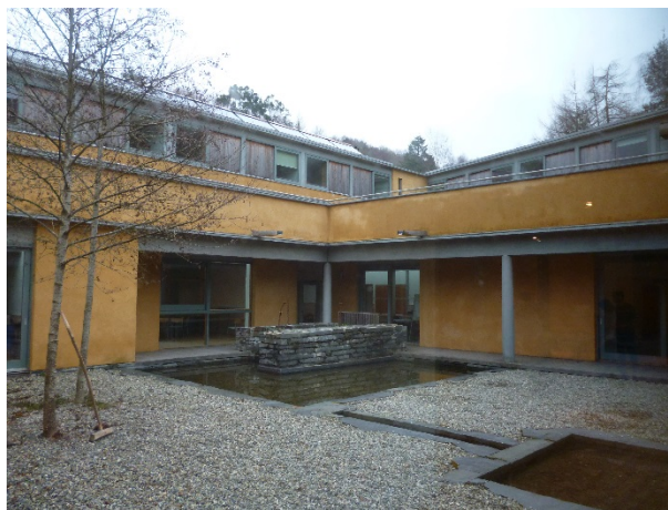
Figure 1.2: The WISE building, teaching facility utilising hemp-lime external walls, Centre for alternative Technology, Powys.
