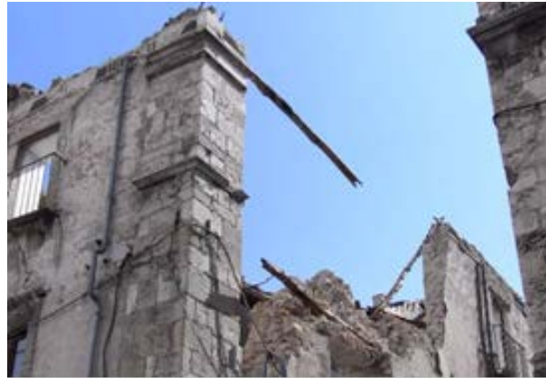
Fig. 2-4: poor performance of timber tie (D'Ayala Paganoni, 2011)
