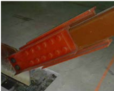
Fig. 2-8: Single bracing Pall's friction damper (Chang et al., 2006)
