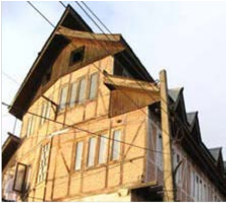
Fig. 2-3: Dhajji-dewari system (Paikara and Rai, 2006)
