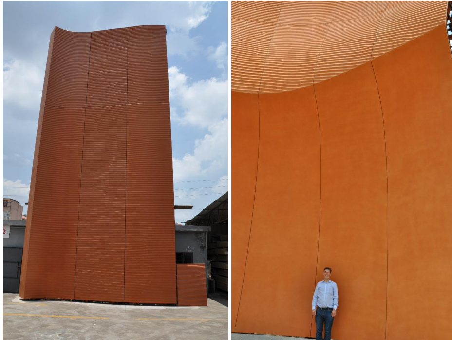
Figure 4-5: Mock up of exterior and canyon panels for the pavilion. Source Foster + Partners.
