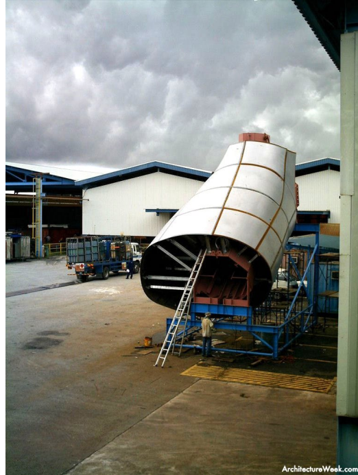
Figure 3-14: Sidra Trees project by Arata Isozaki, showing initial desired image, and resultant optimised structural section in red, and aesthetic cladding in white, images from [Smith, 2007].
