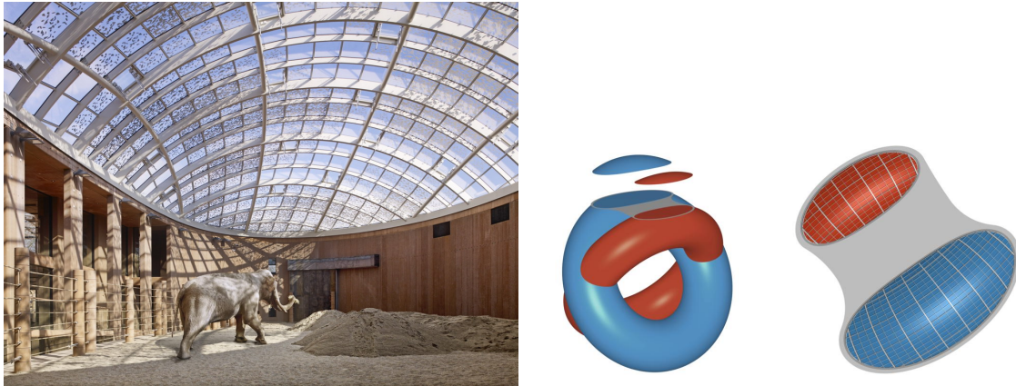
Figure 3-9: The Copenhagen Elephant House, an example of typical pre-rationalised design by Foster + Partners. Using two torus patches as generating geometry, a roof with efficient planar quadrilateral panellization with constant curvature beams can be generated. From [Peters, 2008].
