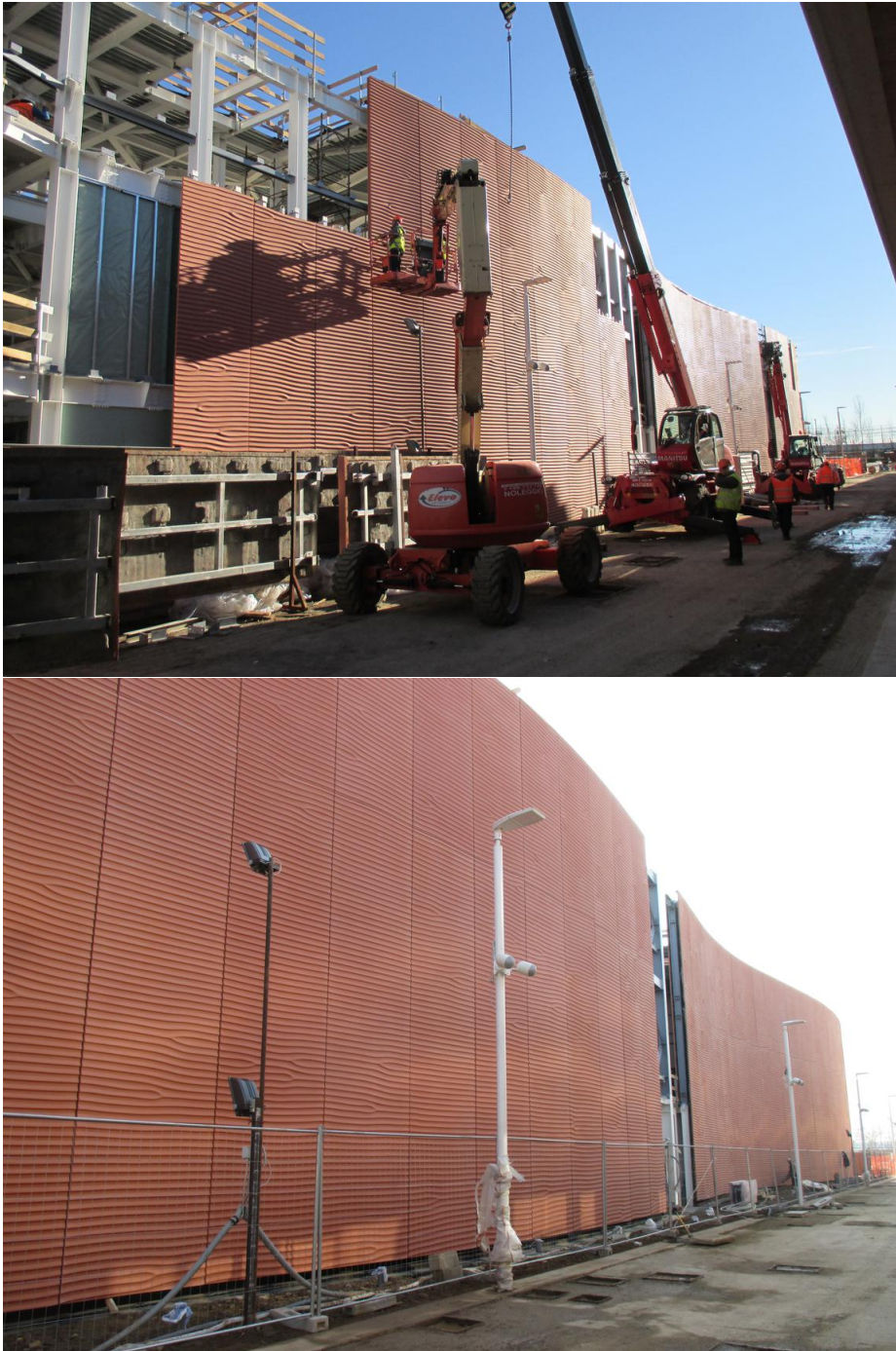
Figure 4-7: Installation of one elevation of panels. Source Foster + Partners.
