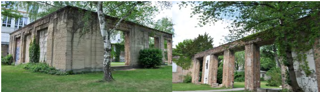
Figure 5. The site for the demonstration project: the gallery at the rear of the University of the Arts in Berlin
