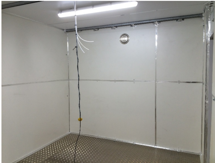
Figure 7.3 PC panels installed on 4 walls of the 30 m 3 chamber.
