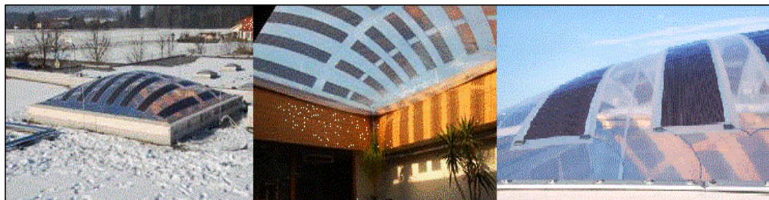
Figure 2.9: Flexible photovoltaic construction integrated in an ETFE cushion (Cremers, 2009)
