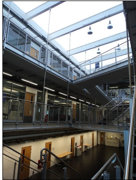
Figure 6.2: ETFE cushions covering the central atrium as viewed from the building interior
