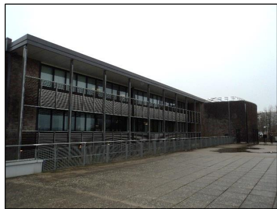
Figure 6.4: South façade of the East Building
