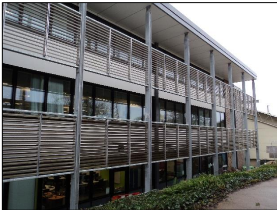
Figure 6.3: West façade of the East Building
