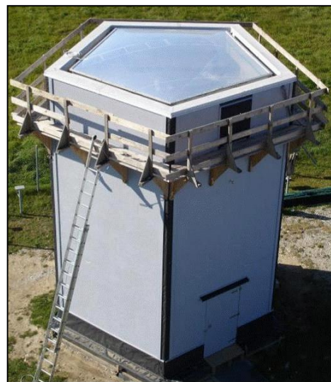
Figure 3.6: Experimental structure with ETFE roof built by the Fraunhofer Institut für Bauphysik (Antretter et al. , 2011)
