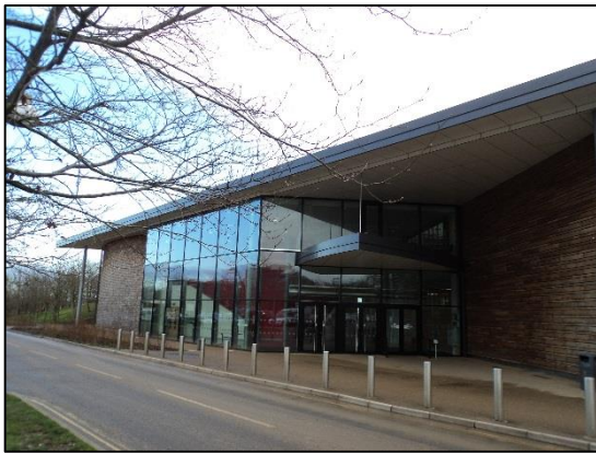
Figure 6.1: North façade of the East Building, main entrance to the building
