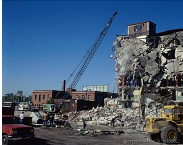
Figure 185 Application of wrecking ball
