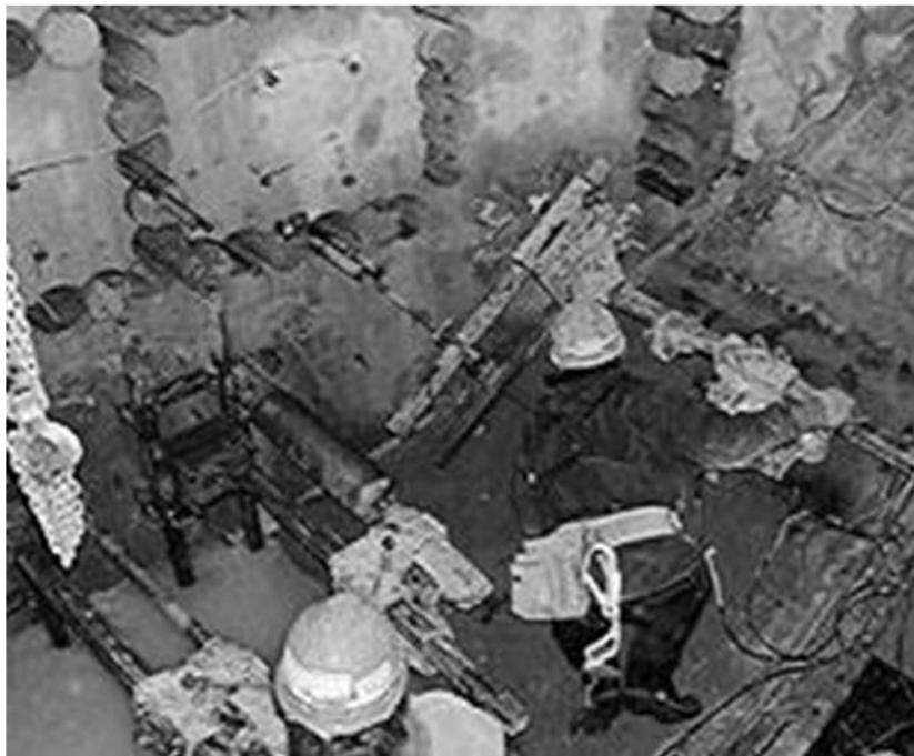
Figure 150 Diamond boring drill application to element cutting (source: Japan Concrete Cutting Industry Osaka Ltd., 2013)
