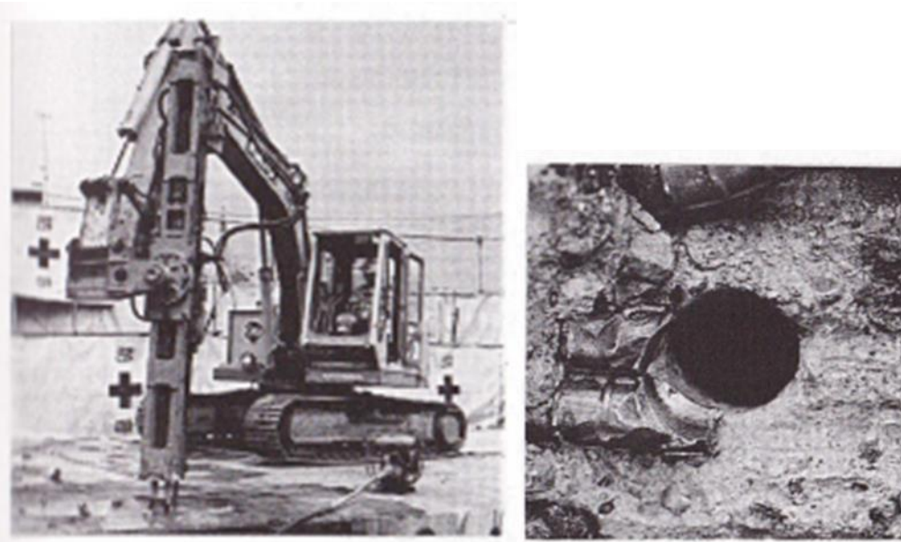
Figure 148 Silent Drill and bored hole
