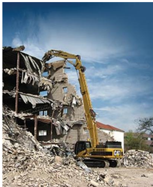
Figure 186 Application of hydraulic breaker
