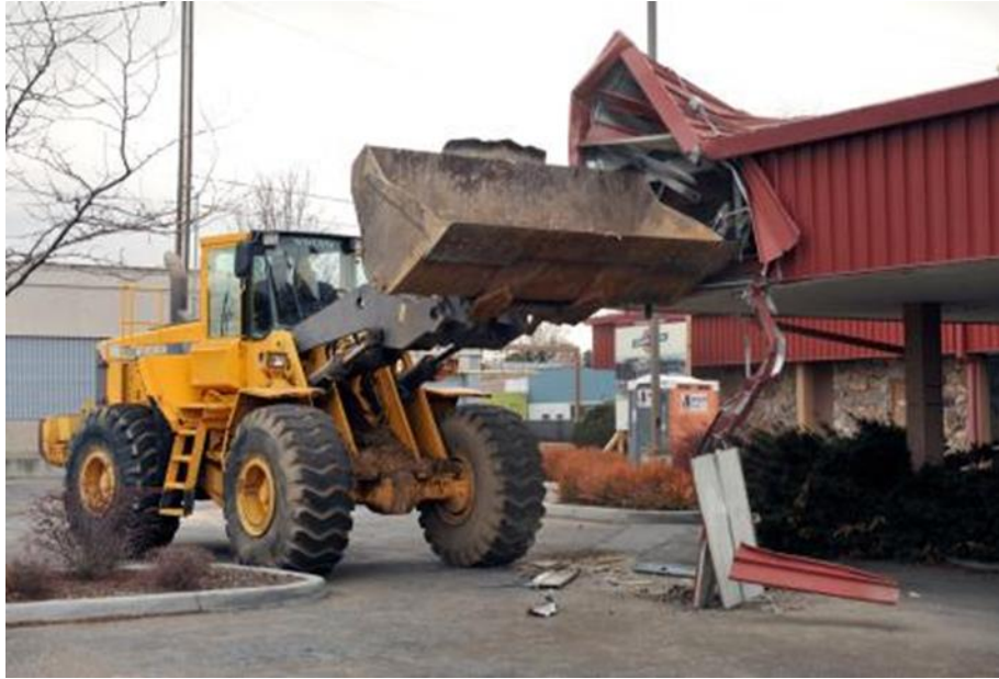
Figure 191 Application of bucket
