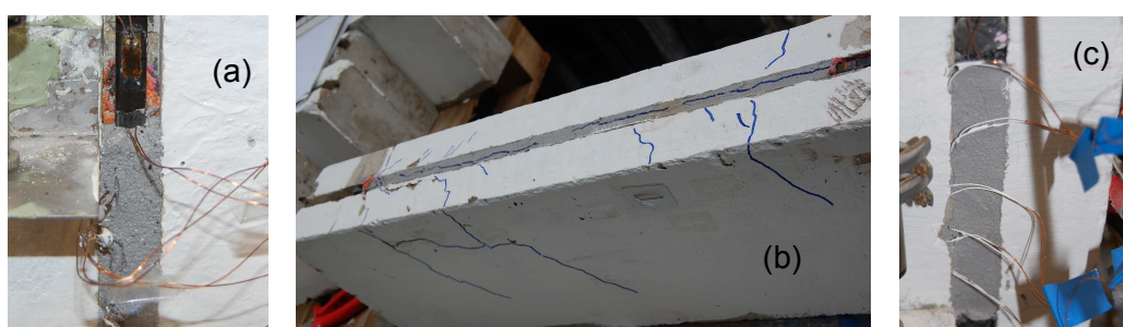
Figure 4.16 - (a) Pull-out failure in specimen 10-39[S/60/L/Sika/6.4p]repeat , (b) pull-out failure accompanied by splitting of the resin cover and the concrete in specimen 9-36[S/60/S/Sika/12.7p] and (c) pull-out failure accompanied by splitting in the concrete with no visible cracks in the resin cover in specimen 10-38[S/60/L/Sika/3.2p]
