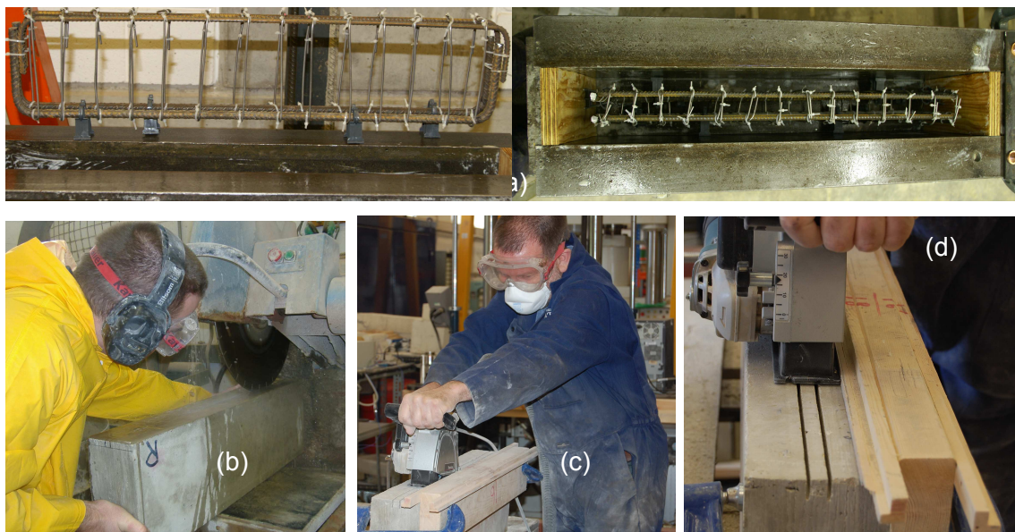
Figure 3.12 - (a) Reinforcement cages, (b), (c) and (d) saw cutting of the grooves on the concrete cover
