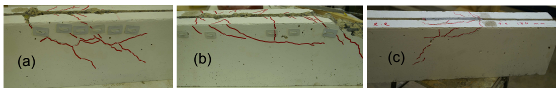
Figure 4.8 - Flexural/shear cracking in specimens: (a) 5-7[C12/30/S/6.4p], (b) 5-8[C12/30/S/12.7p] and (c) 6-15[A9/30/S/6.4p]
