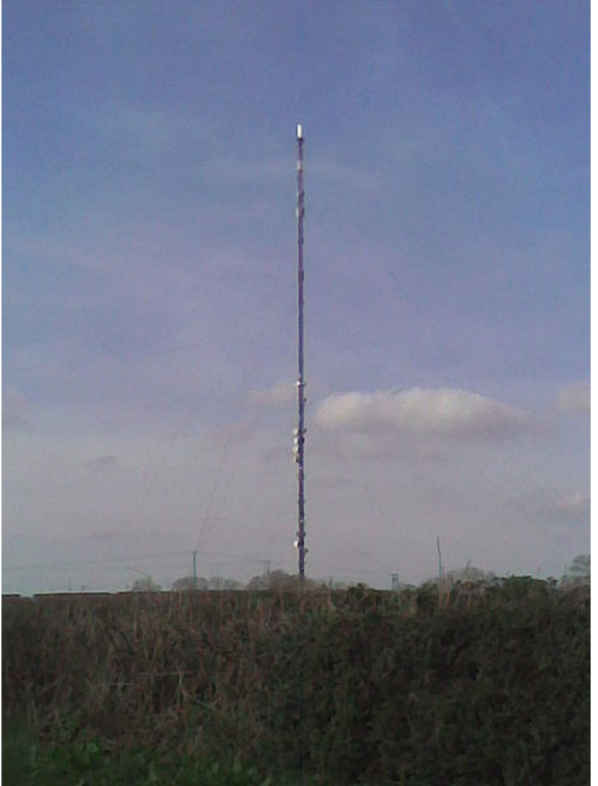
Figure 4-18: Stockland Hill transmitting station. lat. 50.80716 , long. - 3.104809., Height of mast 235 m. 139 Image source Wikipedia, copyright public domain
