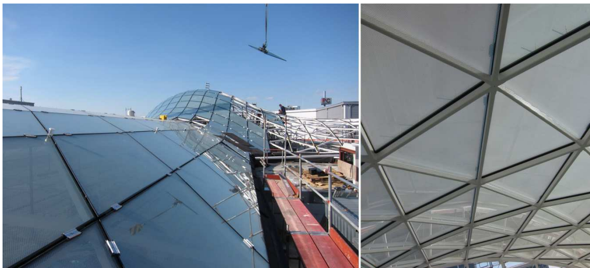
Figure 3 Building envelopes. Left: Translational surface from quadrangular glass panels. Right: Free-form surface built from triangular glass panes. Images courtesy of Schlaich Bergermann and Partners, co-designed by the author.
