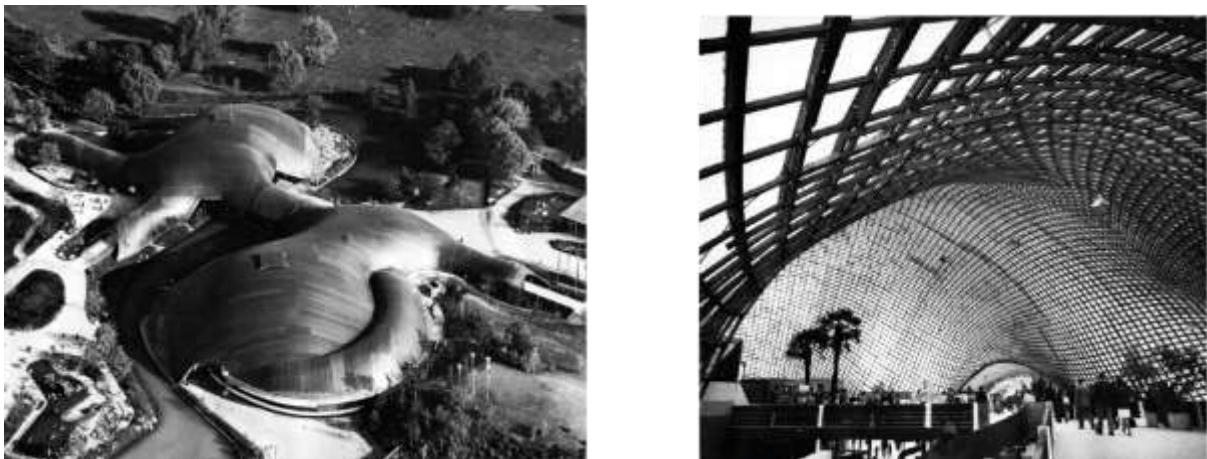
Figure 1. 11 Mannheim gridshell. Left: Aerial view. Right: Internal view. (SMDArquitectes)
