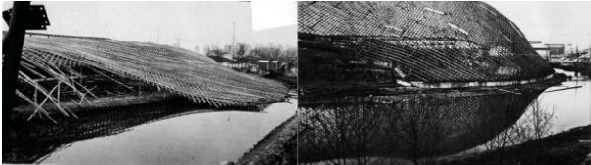
Figure 1. 23 Mannheim gridshell construction. Lifting into shape. (SMDArquitectes)
