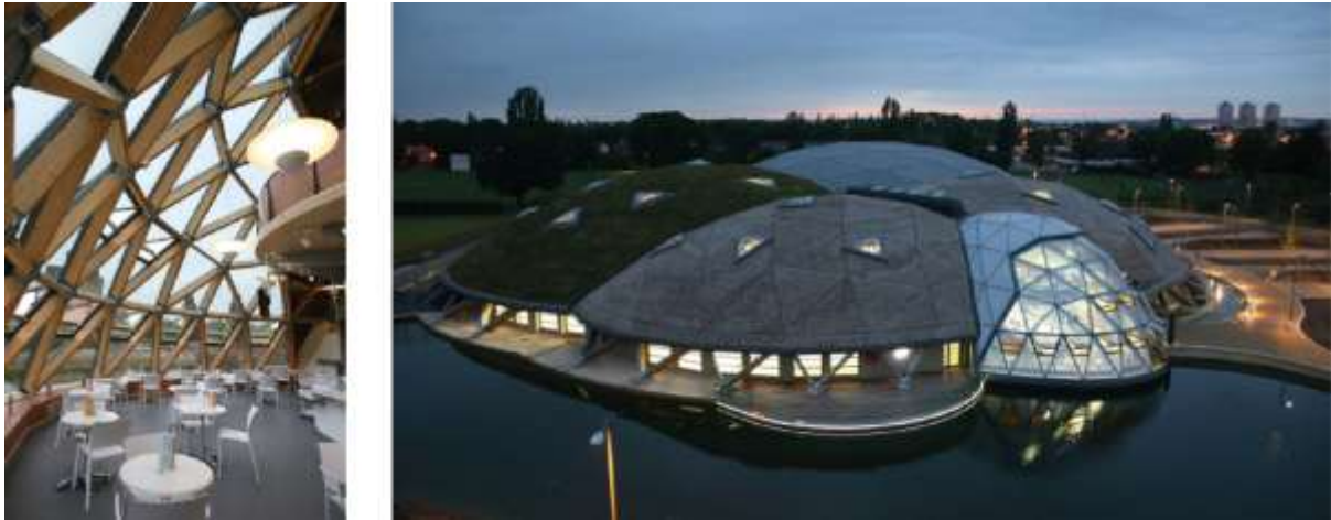
Figure 1.3 Discrete timber member gridshell. Pods Sports Complex (S&P Architects)
