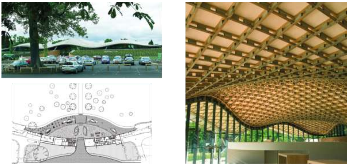
Figure 1. 16 Savill Garden gridshell. Top-left: External view. Bottom-left: Plan. Right: Internal view. (Architect’s Journal)
