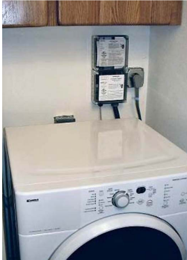
Fig. 2.14 Domestic demand response module installed on a washing machine
