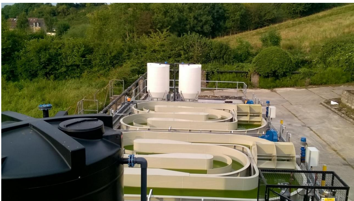
Figure 6.1: Pilot-scale HRAPs in Beckington WWTPs managed by the University of Bath, where Av_12 was applied for secondary effluent WW treatment.
