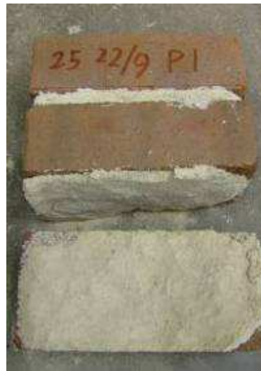
(b) Mortar failure
