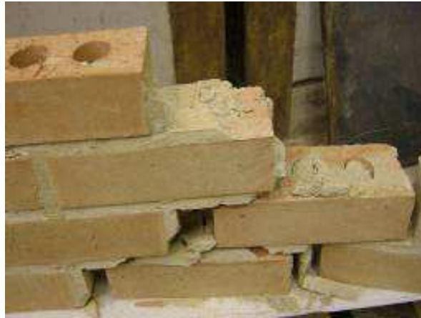
Figure 5.8 Mortar splitting in brickwork using 'Hardwicke Welbeck Autumn Antique' brick
