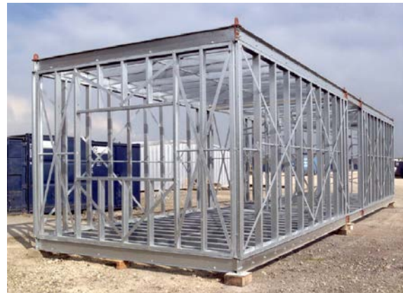
Figure 2. Light steel framework of a module
