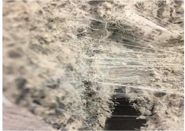
Figure 1. Close-up showing the fibres in the concrete.
