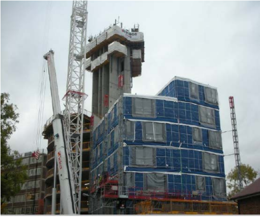
Figure 3. High-rise modular building, Wembley, UK
