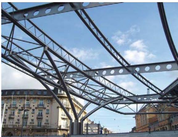
Figure 1. Structural stainless steel at Gent Sint Pieters railway station in Belgium.
