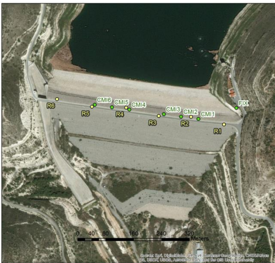
Figure 2: Instrumentation on the dam crest
