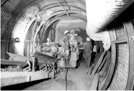
Figure 2. Excavation of TT10 tunnel.
