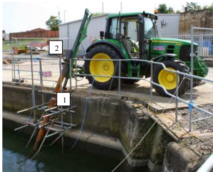
Figure 1. The pile driving set-up used: 1) the steel pipe; 2) post-driver hammer.
