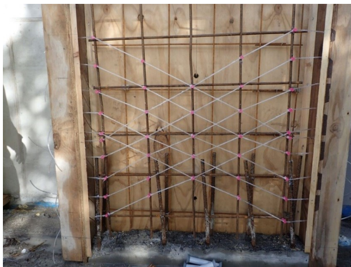
Figure 5 Embedded capillary network installed prior to casting of the concrete
