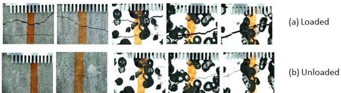
Figure 7 Cracking of the bacteria-based panel: (a) cracks immediately upon loading, and (b) residual cracks after unloading.
