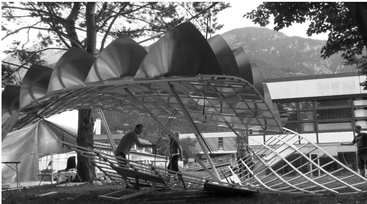
Figure 7: Replacing lashing straps by 4 cables, each starting from a distributor plate and branching out to four nodes on the top grid.
